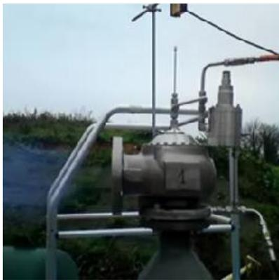
Top : Pressure transmitter and buffer tank on the main valve
